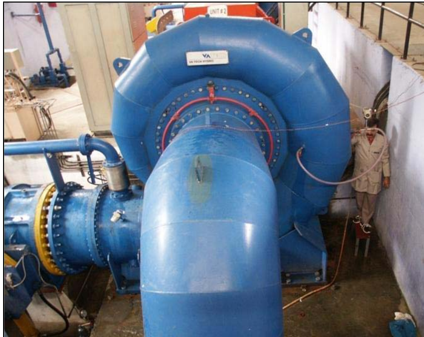
Fig. 28 : Illustration of pressure taps in vertical steel spiral case
