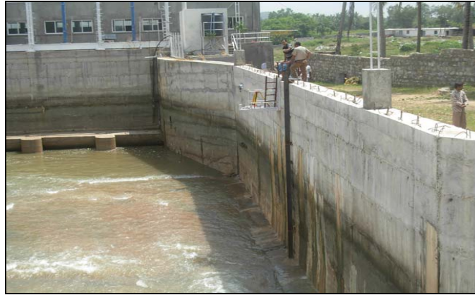
Fig. 24 : Guide rail fixed to the channel wall for guiding movement of ADCP trolley
