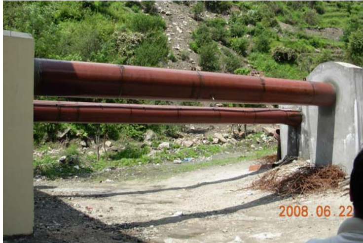
(a) Adequate length of penstock left un-embedded for installing transducers
