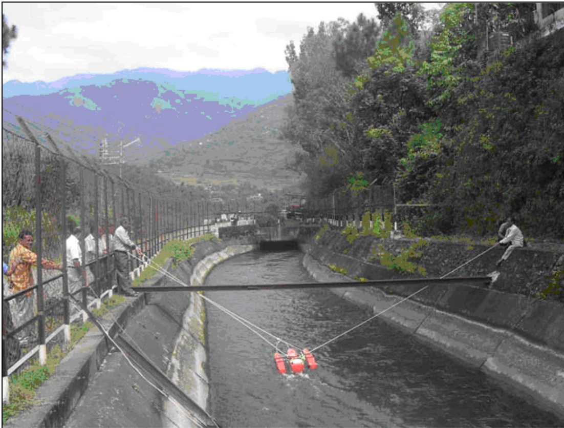
Fig. 26 : Maneuvering V-ADCP from channel banks
