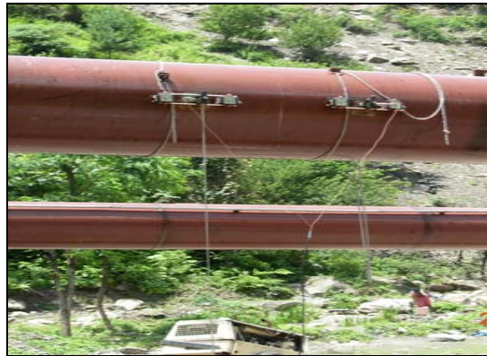
(b) Transducers of UTTF clamped on a penstock in reflection mode
